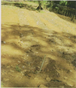
Figure 04 – Preparation of trenches
